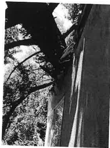
Tree remaining on west unit of 8-plex
