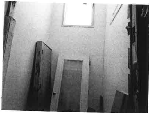
Removed spiral staircase
