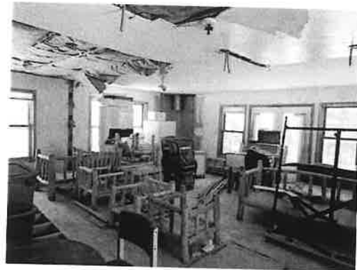
Upper level of former manager's quarters
