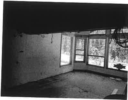
First level of lodge/office
