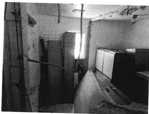
Gutted restroom in upper level
