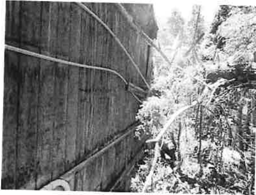
West wall of 8-plex
