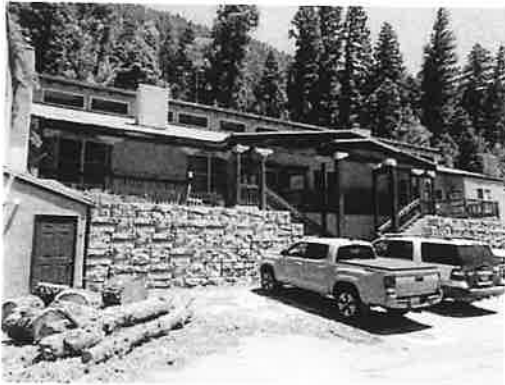
Rear elevation of 8-plex
