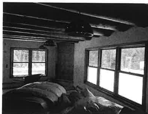
Interior of first level of former lodge/office
