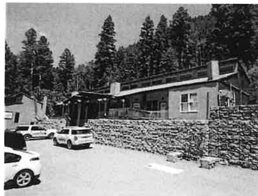
Front elevation of 8-plex
