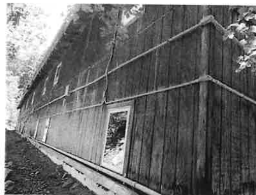
Rear elevation of 8-plex
