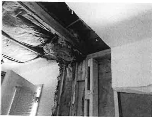
Roof leak
