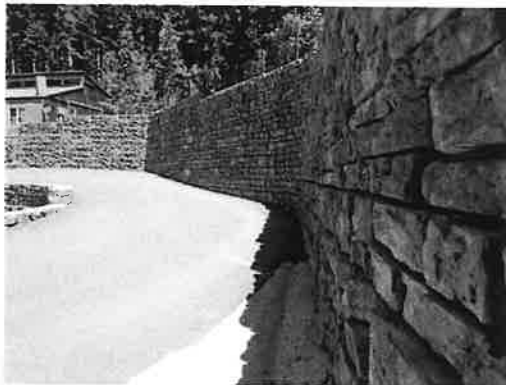
New driveway and retaining wall
